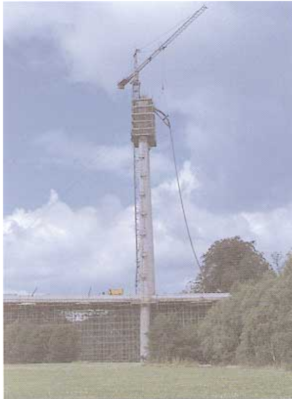
◀ Lightness of the 200 SSI cables speeds up erection
