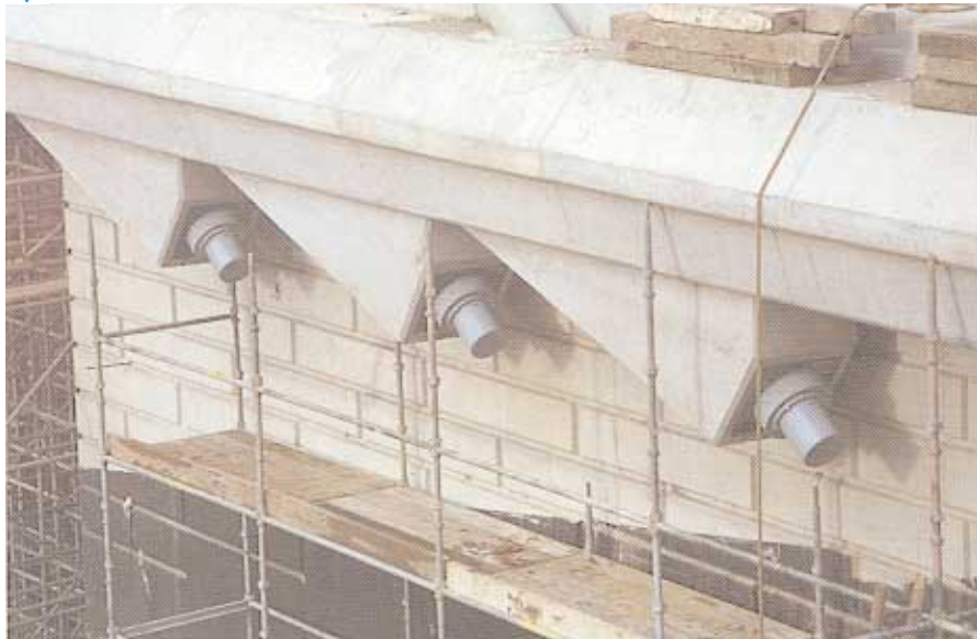
▼ Anchorages are already in place
