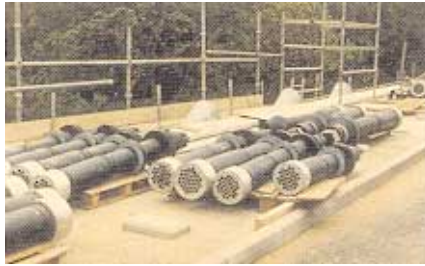
▲ Anchorages ready for erection
